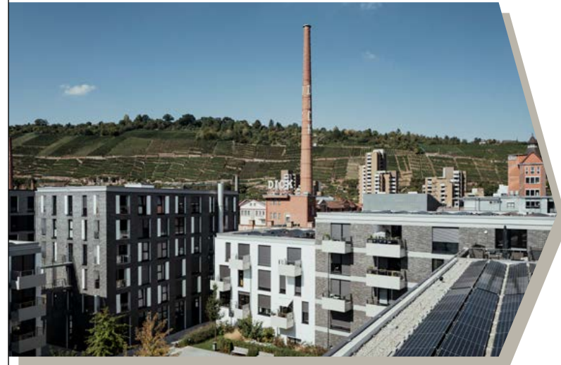
A TOTAL OF 4,200 SQUARE METERS OF PHOTOVOLTAICS HAVE BEEN INSTALLED ON THE ROOFS OF THE RESIDENTIAL BLOCKS, WITH AROUND 10,000 IN THE ENTIRE URBAN DISTRICT.
